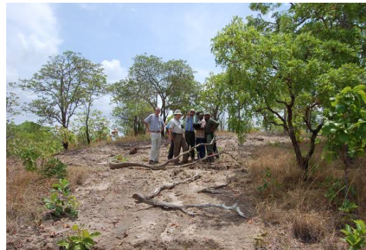
Road rehabilitation at Mantra mineral exploration site
