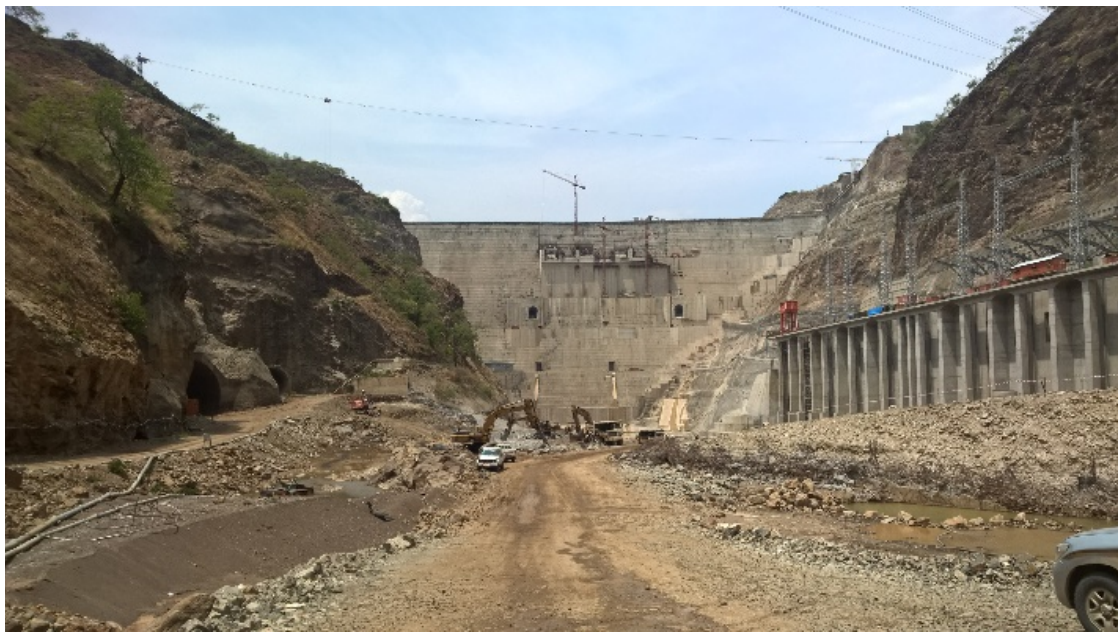
Figure 3. The Gibe III dam and the powerhouse on the right. ©IUCN/E.Saaf
