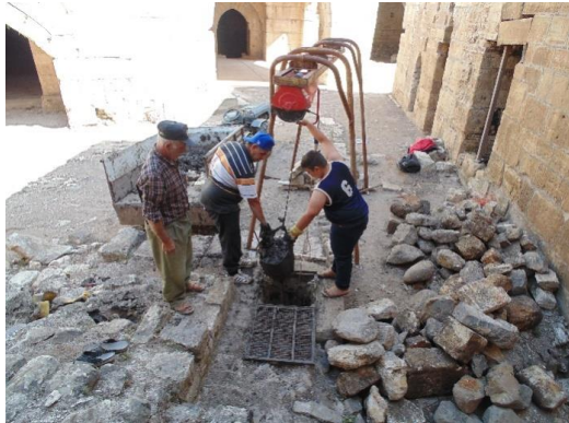
Cleaning the well and removing the debris
